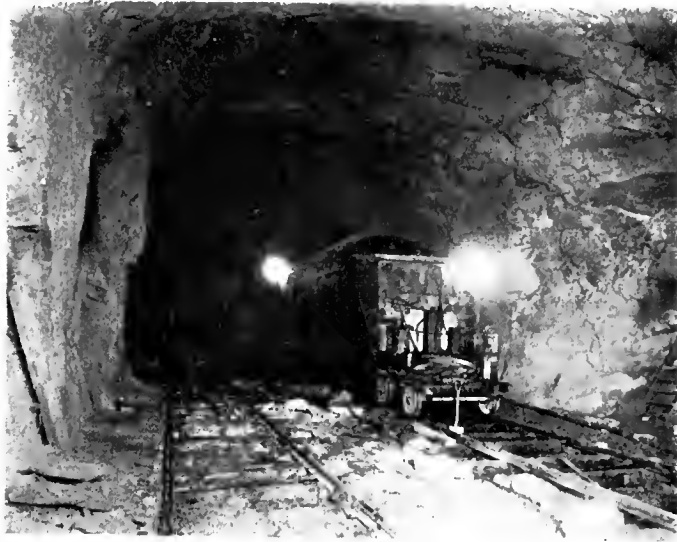
Main Heading Rogers Pass Tunnel—Steam Shovel on standard gauge track at work
